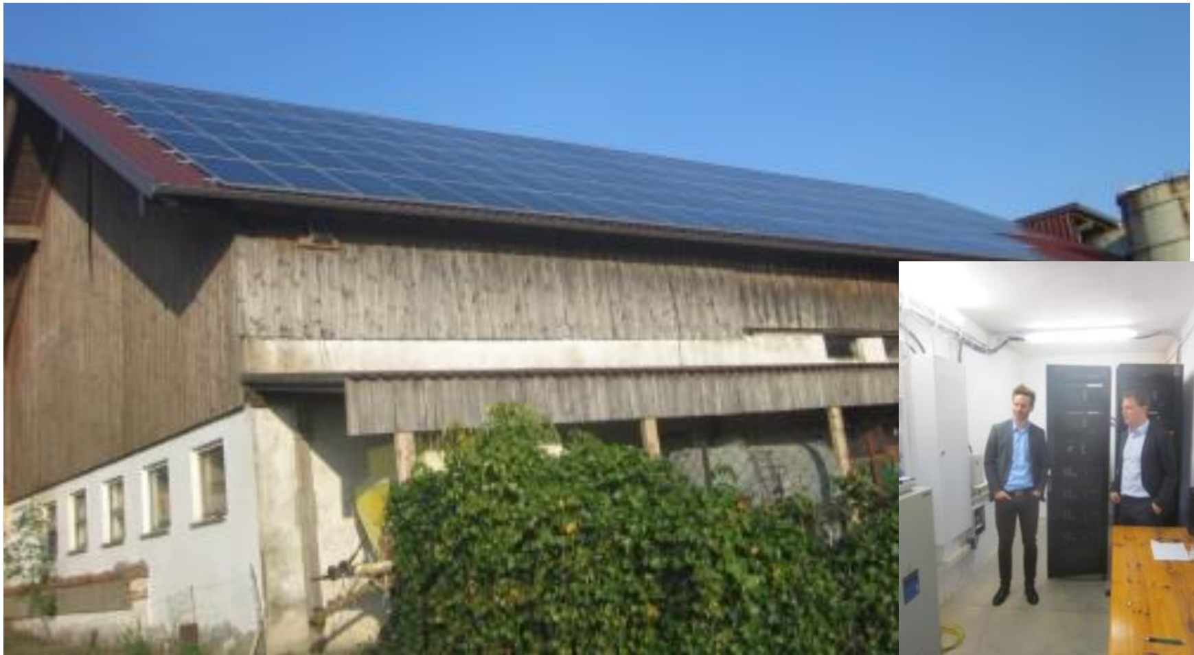
Lagerhaus Feilmeier, COMMERCIAL 40 kW / 45 kWh
